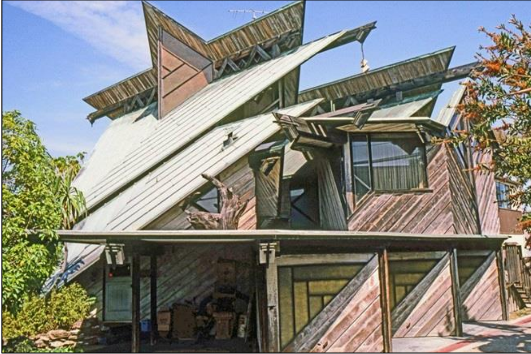
Figure 11 Russell E. and Virgie R. Babcock House at 2694 Bayside Walk, Mission Beach, circa 1959; Source: Kendrick Bangs Kellogg, Facebook
